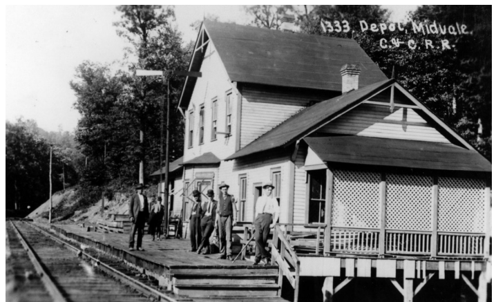
Coal & Coke Railroad Depot at Midvale, Upshur County, West Virginia, ca. 1910.
