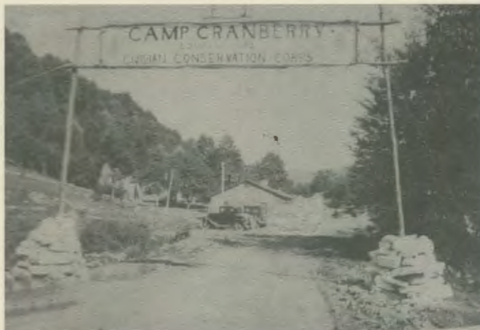
Civilian Conservation Corps Camp Cranberry, Webster County, ca. 1935.
