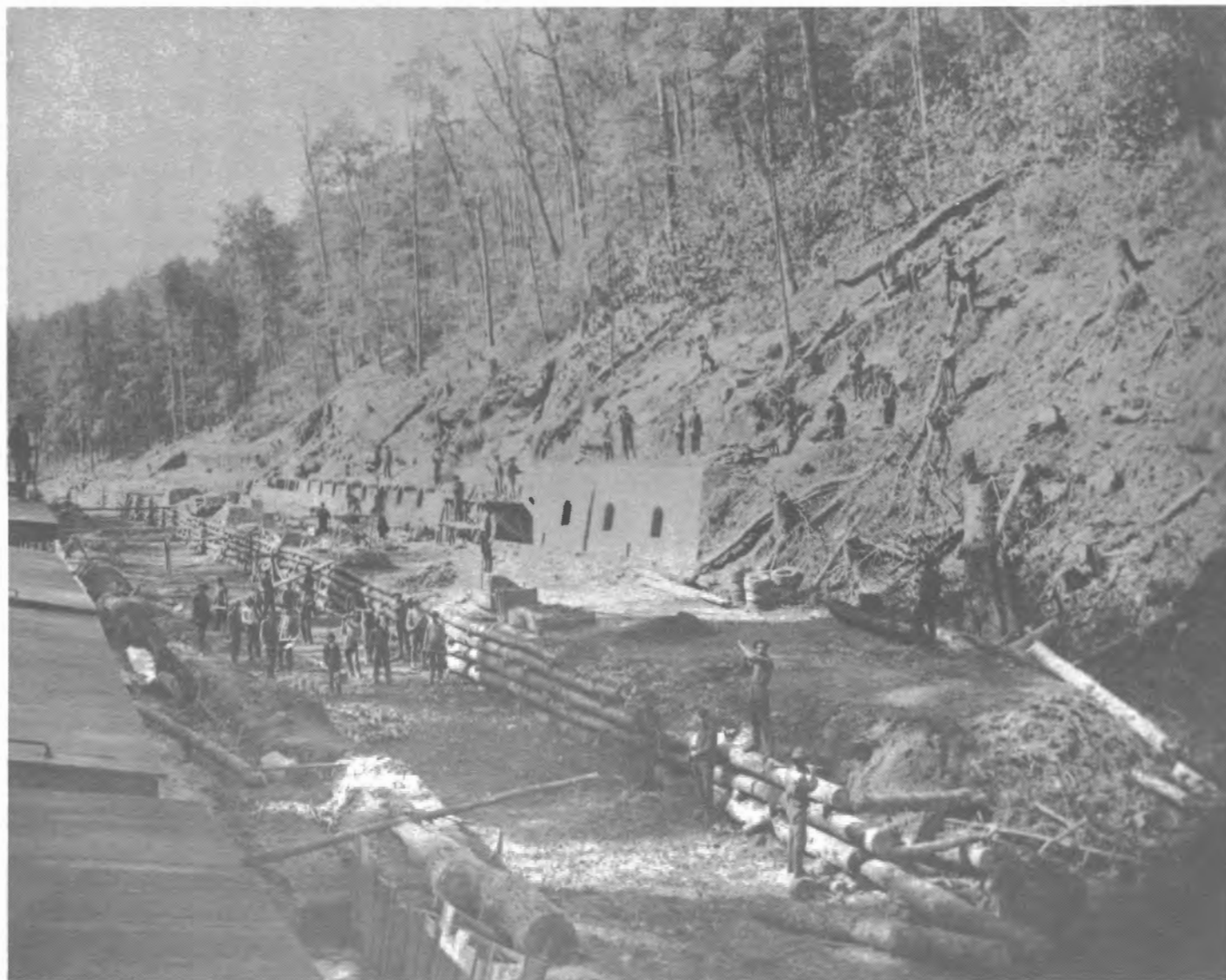
"Erecting Bee Hive Coke Ovens," McDowell or Mercer County, circa 1890.
