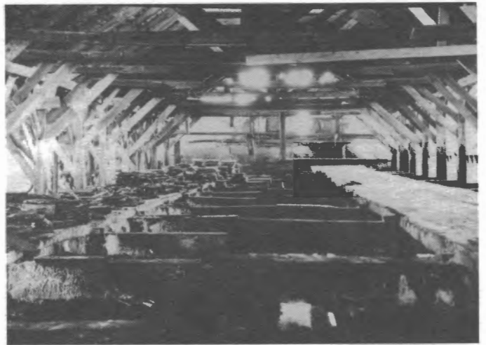
J.Q. Dickinson Company, 1910. Salt was lifted out of the water in these vats and placed on board walkways to dry.
