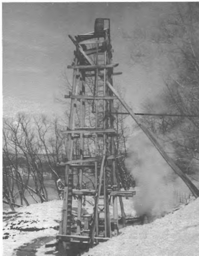
A J. Q. Dickinson Company salt well in operation on the banks of the Kanawha River near Malden, West Virginia, ca. 1910.
