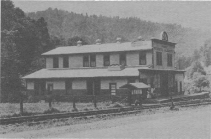
Interior and exterior of Premier Company Store, Pocahontas Collieries Co.
