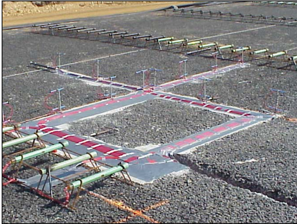
Figure 4.2 Typical Slab Instrumentation Prior to Concrete Placement.
