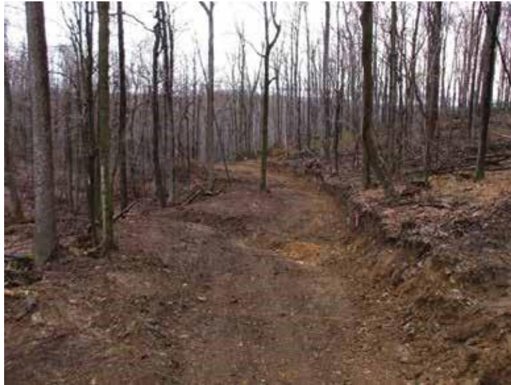
Figure 2. A typical water bar in place on a skid trail.
